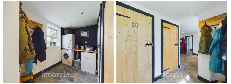
Plumbing for washing machine, spotlights, boiler, wood panel walls, tiled flooring Upvc window.
