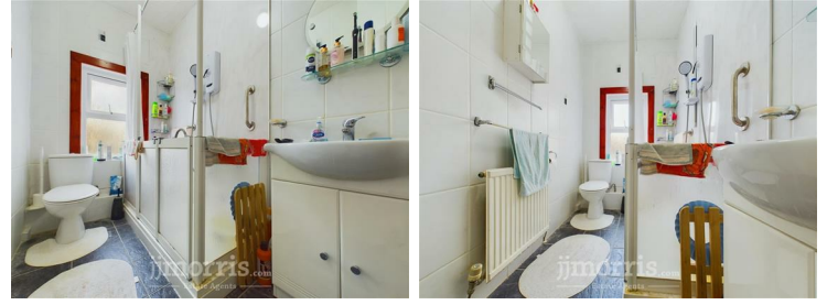
Shower enclosure with electric shower, low flush WC, hand wash basin with unit, tiled walls, tiled floor, Upvc window.
