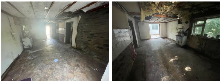
Former Kitchen 20'2" x 12'5" (6.15m x 3.78m)
