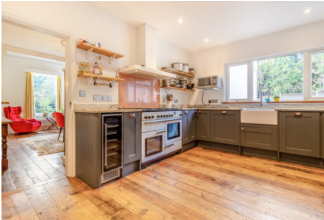
hot water cylinder.
