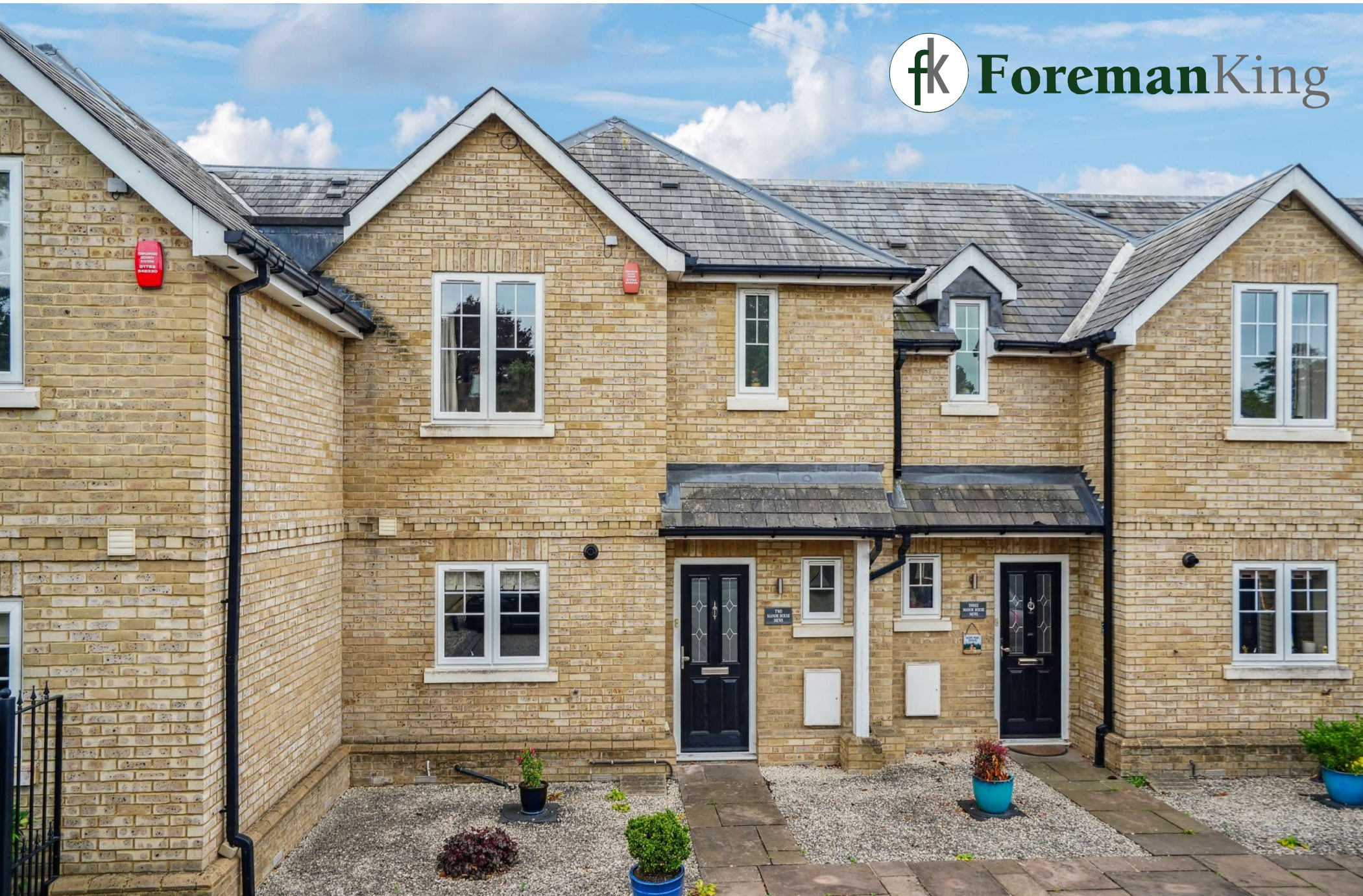
2 MANOR HOUSE MEWS, KINGSWAY, FARNHAM COMMON, BUCKINGHAMSHIRE, SL2 3ST - £730,000 FREEHOLD
