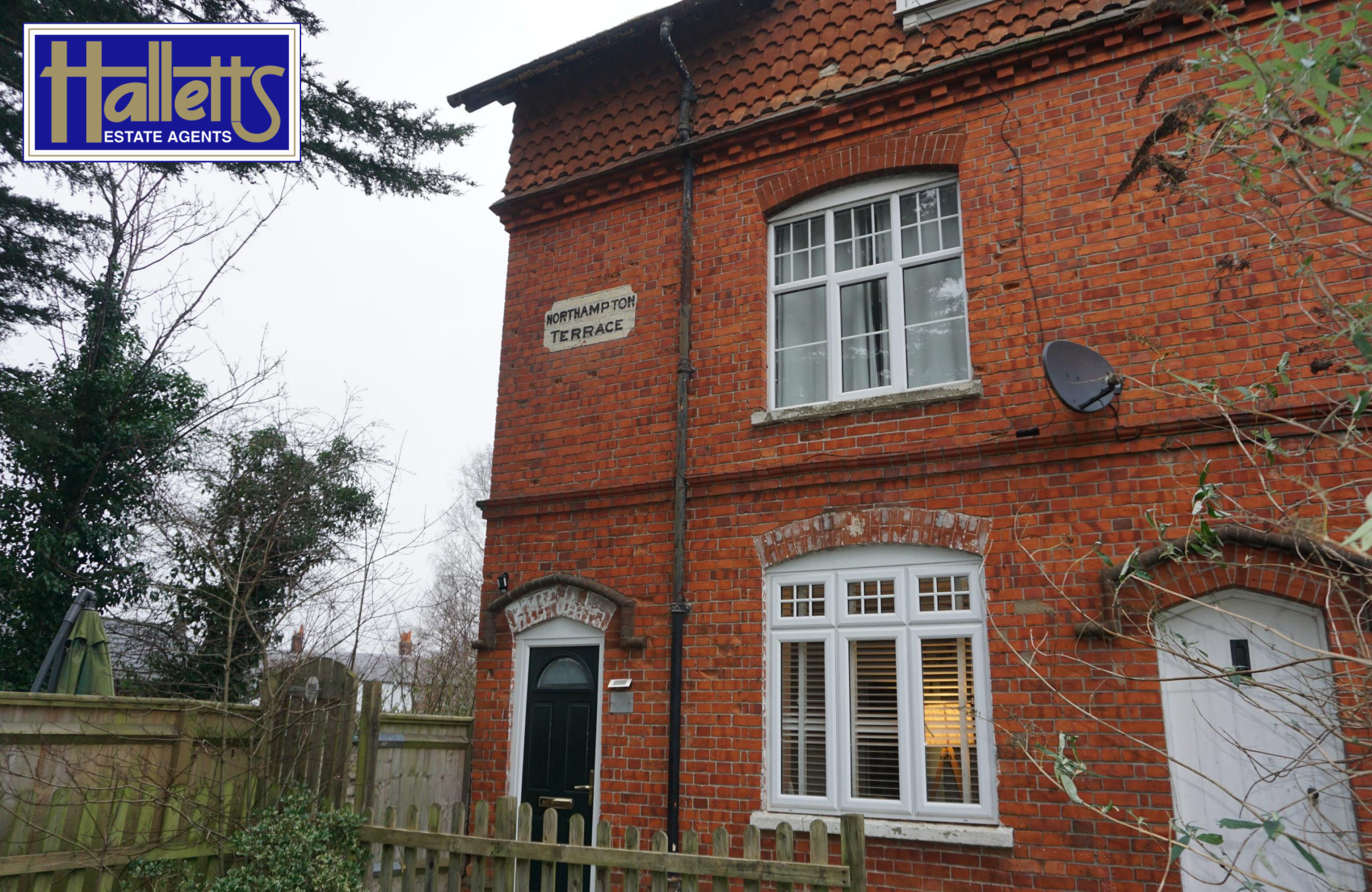
Northampton Terrace 118a London Road Newbury Berkshire RG14 2AJ
