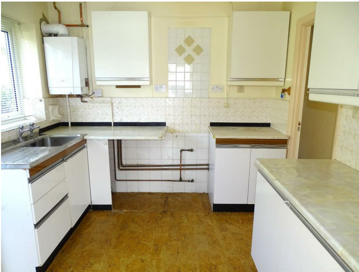
KITCHEN (needs refitting)
