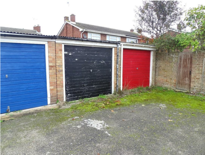
GARAGE IN BLOCK TO REAR
