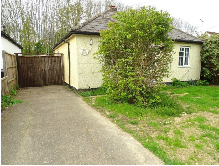
DRIVEWAY TO SIDE
