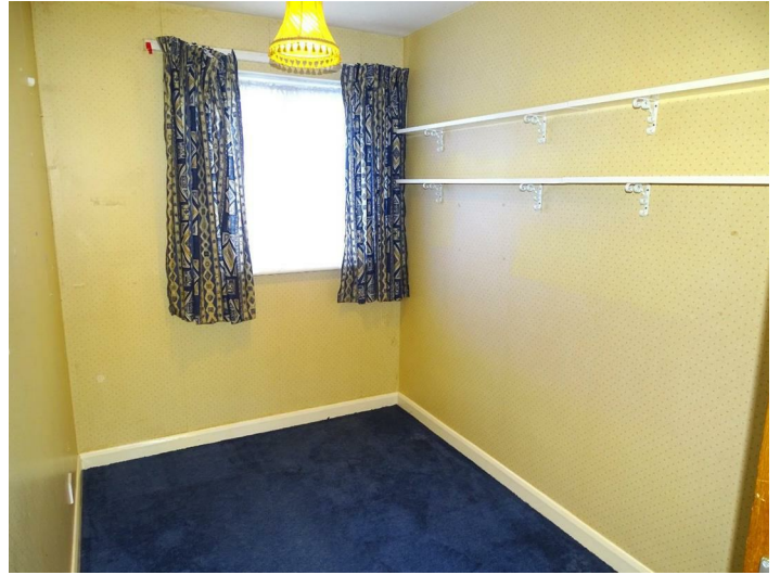
Over stair cupboard, upvc double glazed window.
