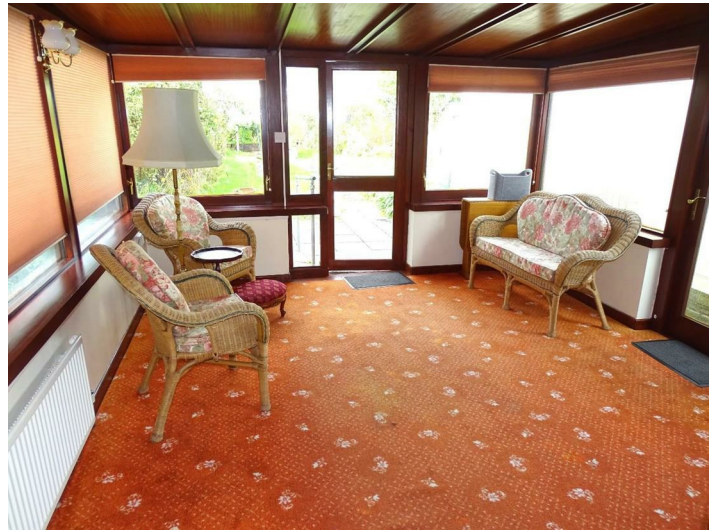
Brick built with wooden double glazed windows and separate double glazed doors to rear garden.
