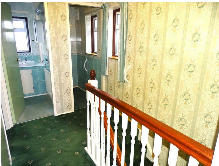
Access to roof space (not boarded), airing cupboard, double glazed window to side.
