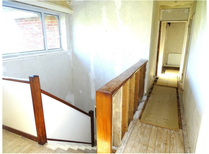
Radiator, upvc double glazed window to front, access to roof space, recess with hot water cylinder (NOT TESTED).
