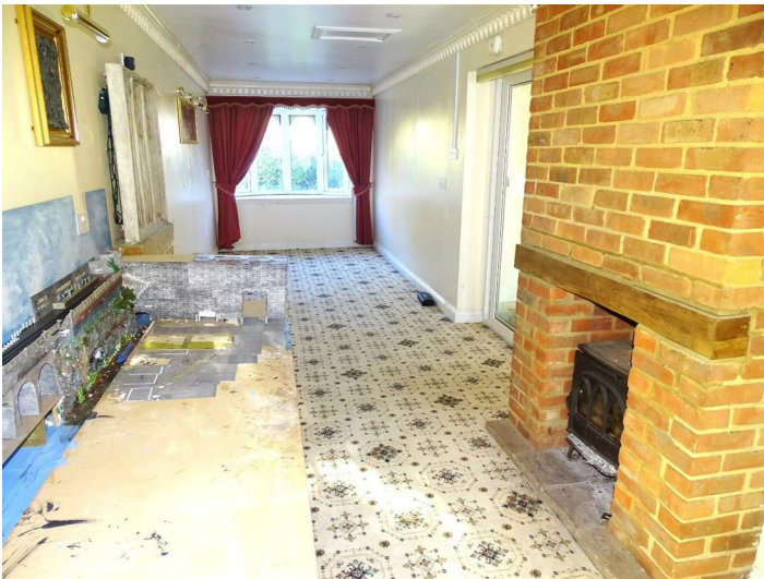
Floor to ceiling brick fireplace, bay upvc double glazed window to front.
