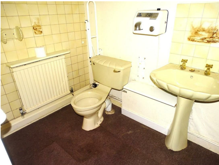
Radiator, low level wc, pedestal wash hand basin.
