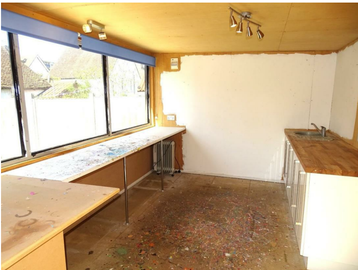
ELECTRICS AND PLUMBING CONNECTED
