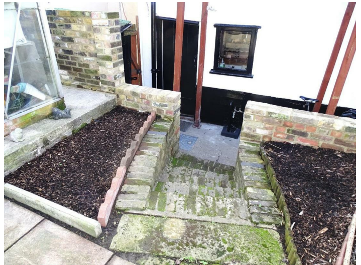
STEPS DOWN TO KITCHEN DOOR
