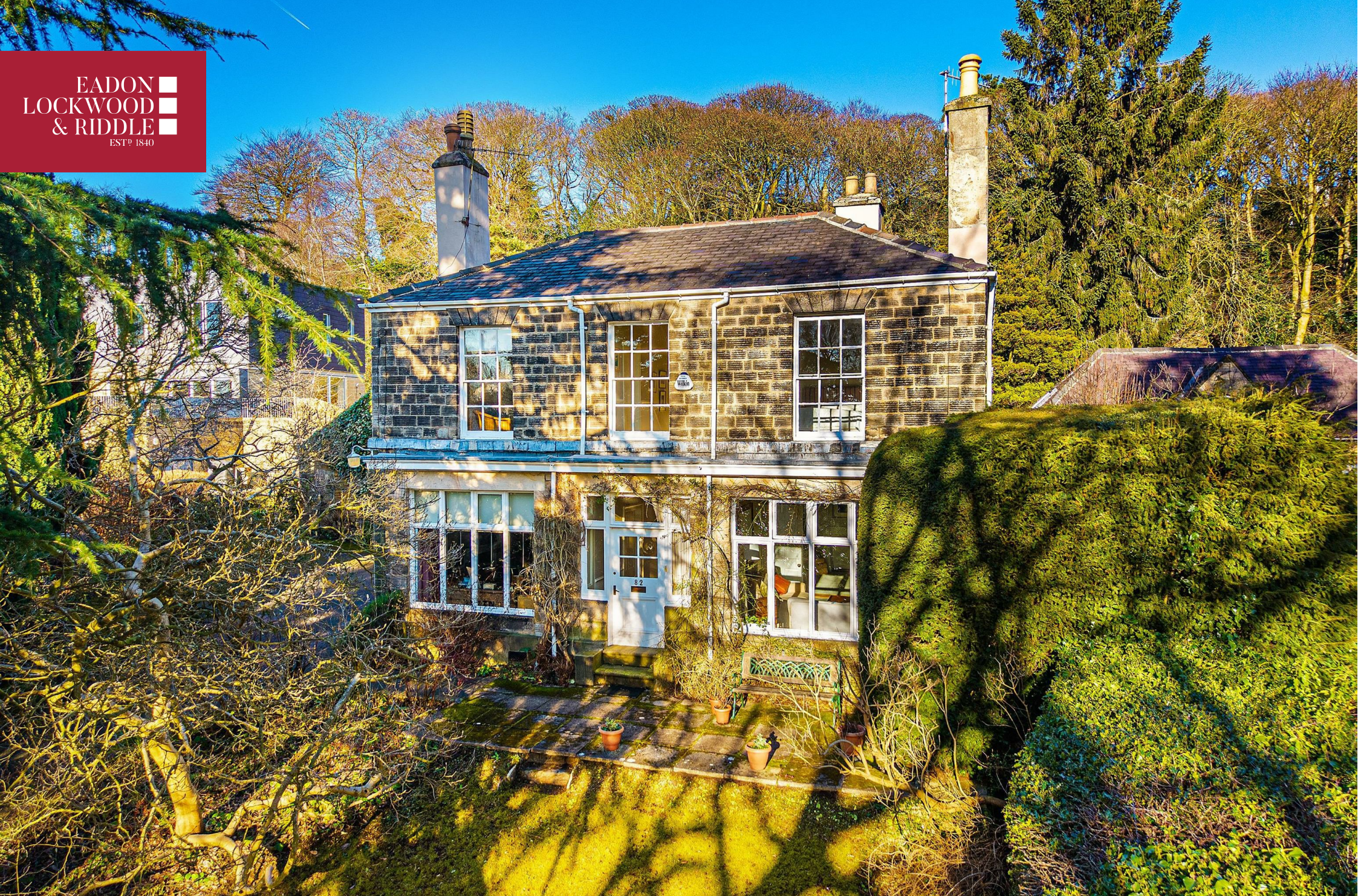
Cliffe House, 82 Ranmoor Road, Sheffield, S10 3HJ
