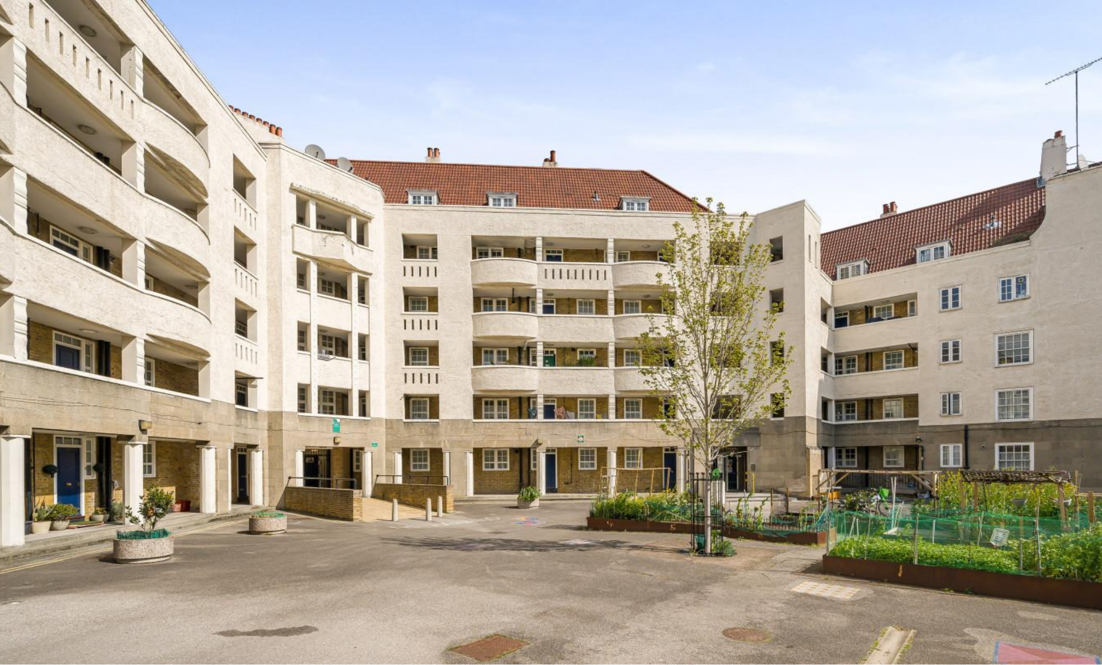
Levita House, Chalton Street, London NW1
