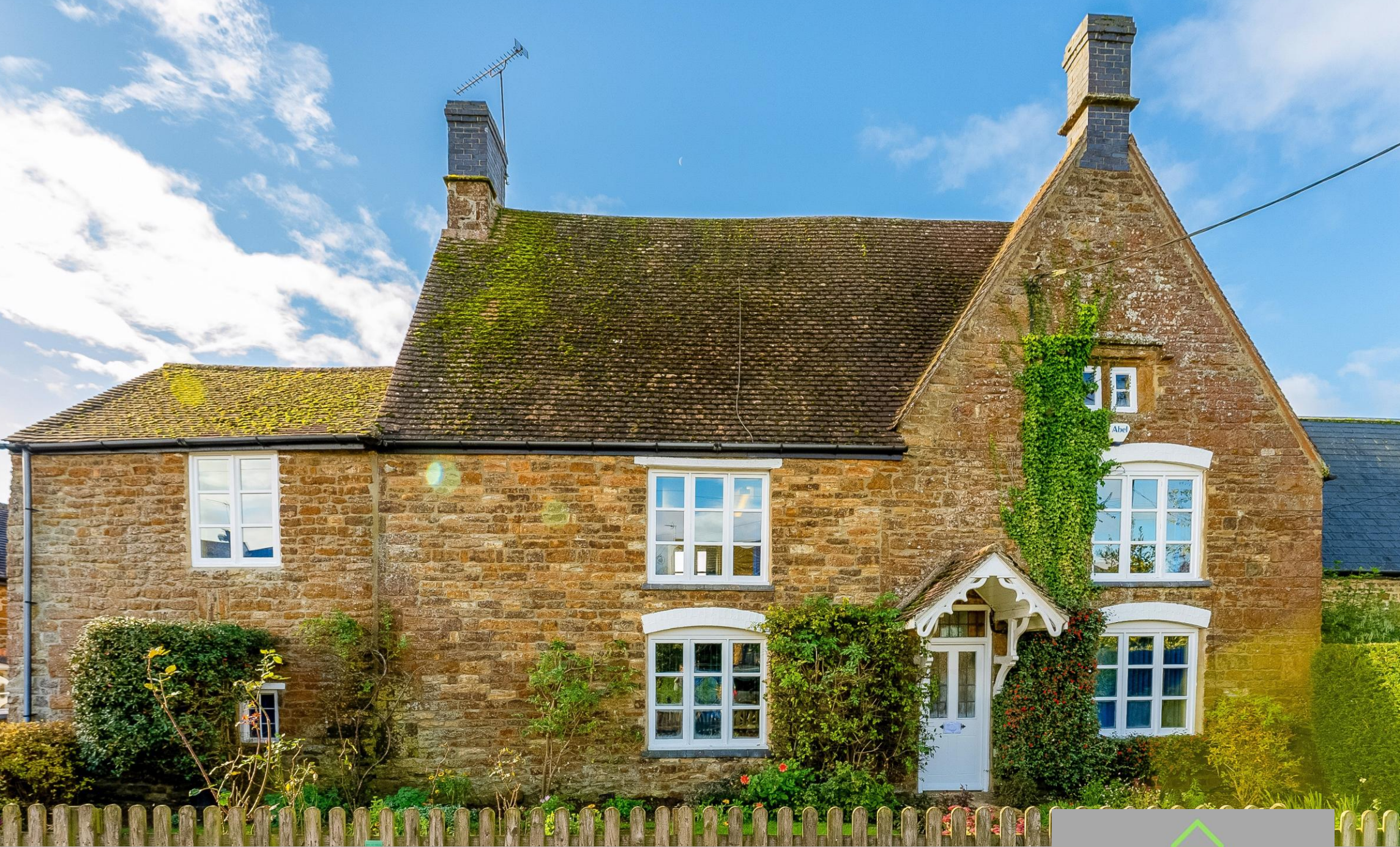
Middleton Farmhouse Main Road, Middleton Cheney
