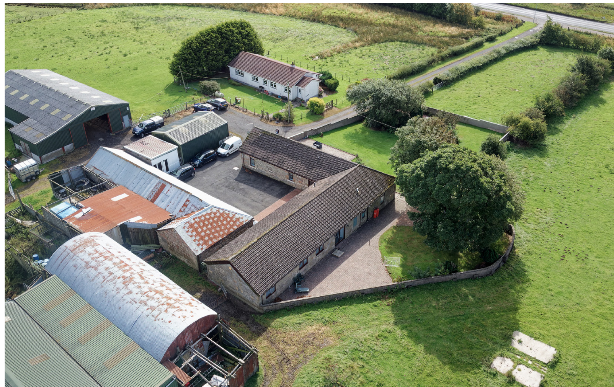
2 PEATPOTS FARM - NEWHOUSE, NORTH LANARKSHIRE
