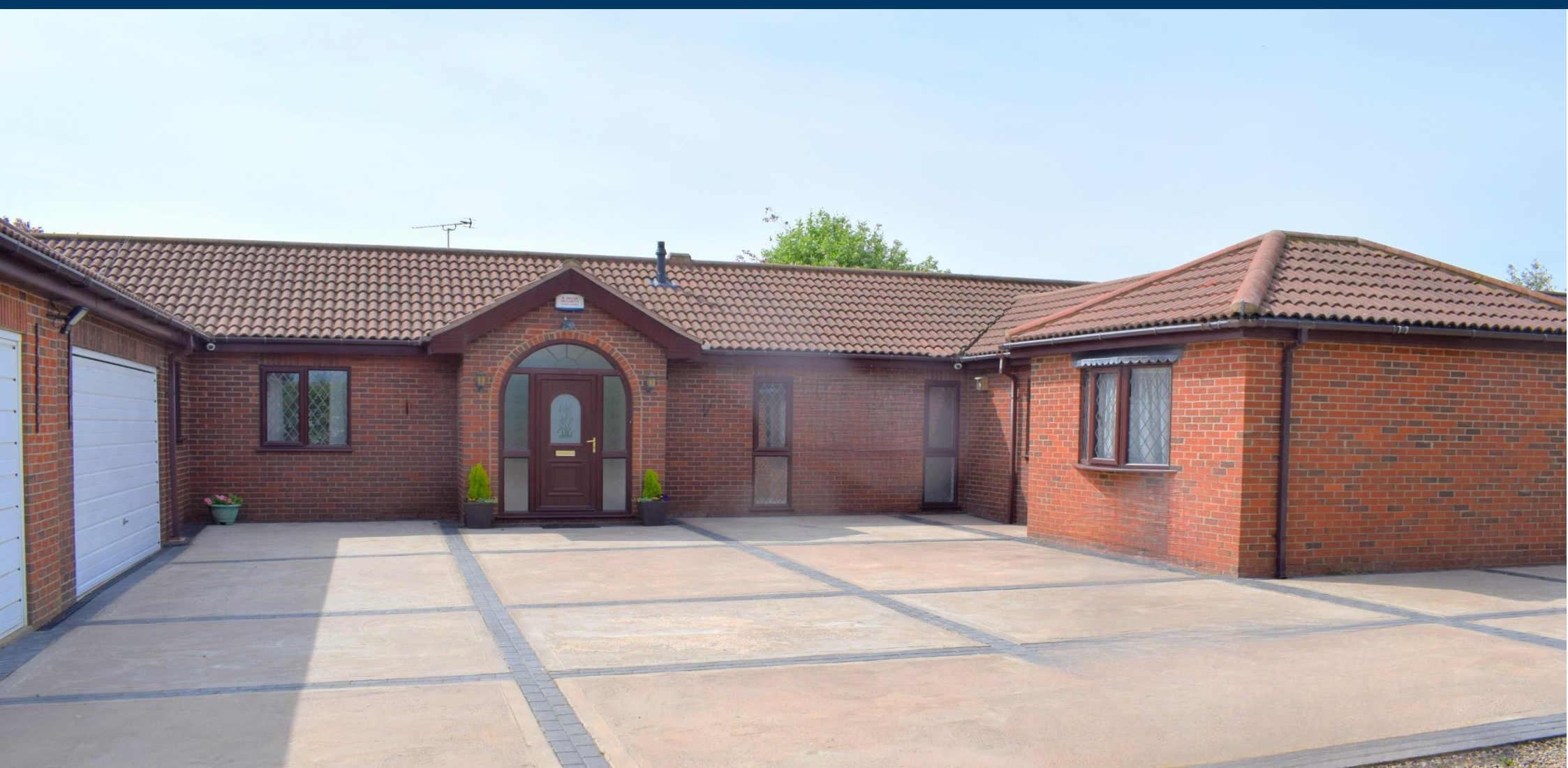
Cottage Close, Hibaldstow
