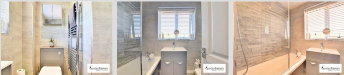
Modern suite featuring a low level WC, washbasin vanity
