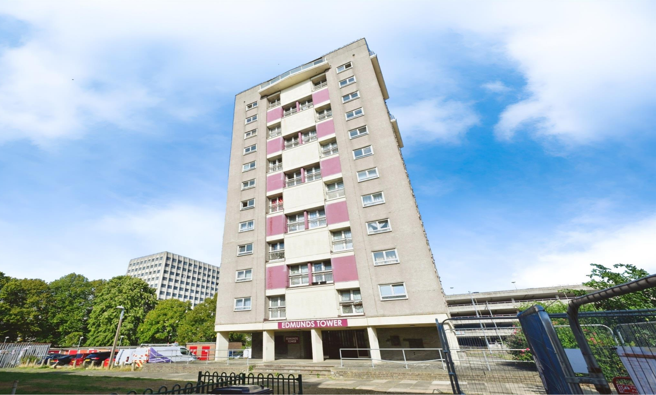
Edmunds Tower, Harlow CM19 4AD
