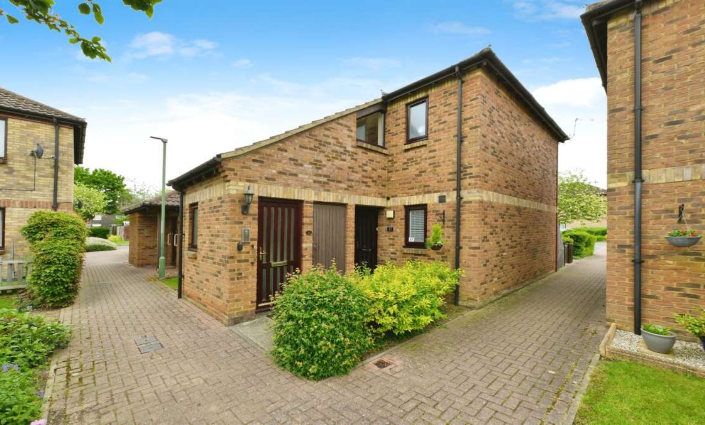
Southern Lodge, Harlow CM19 4NH
