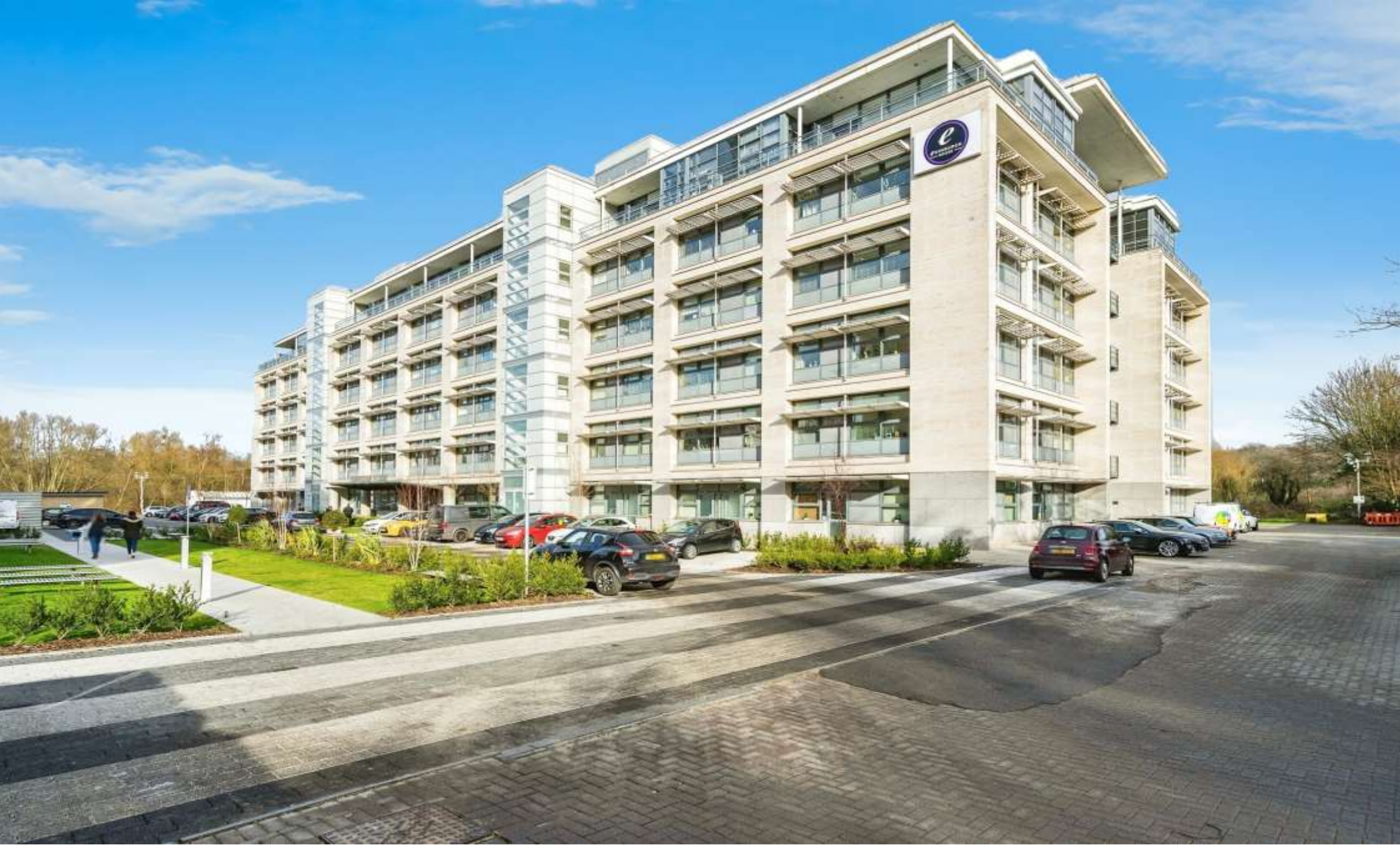
Edinburgh House Edinburgh Gate, Harlow CM20 2JE
