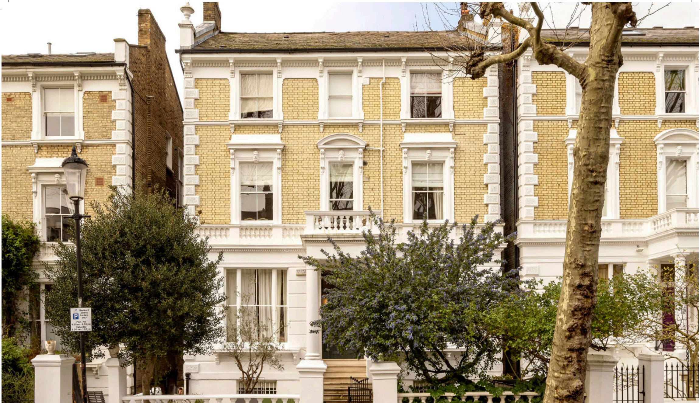
Bassett Road, Notting Hill W10
