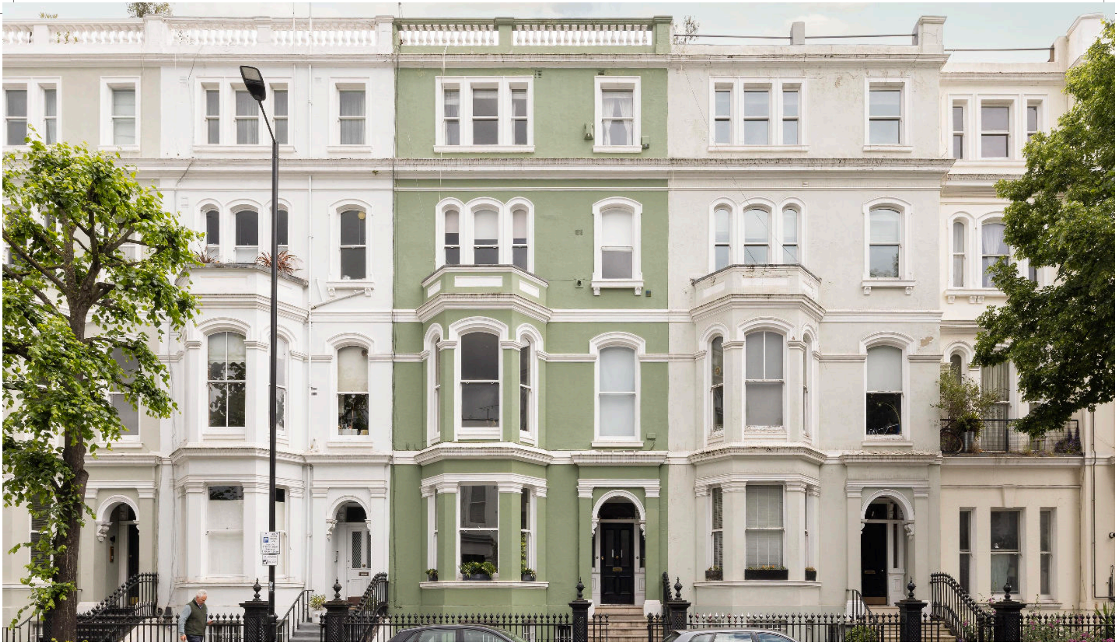
Ladbroke Grove, Notting Hill W11
