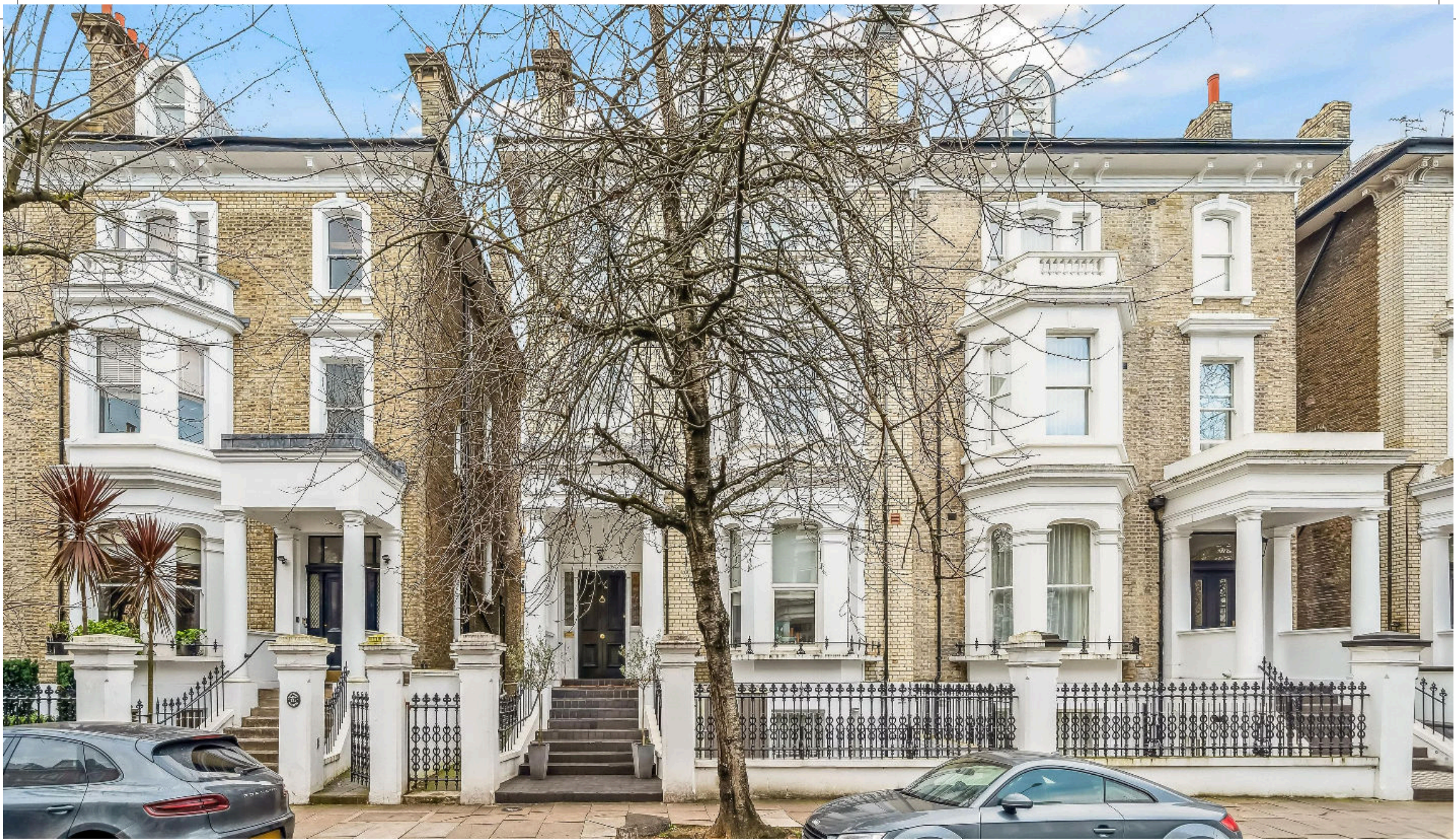
Redcliffe Gardens, London SW10
