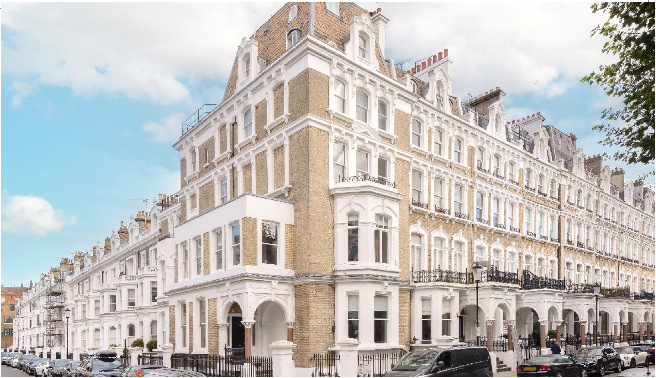
Redcliffe Square, London SW10
