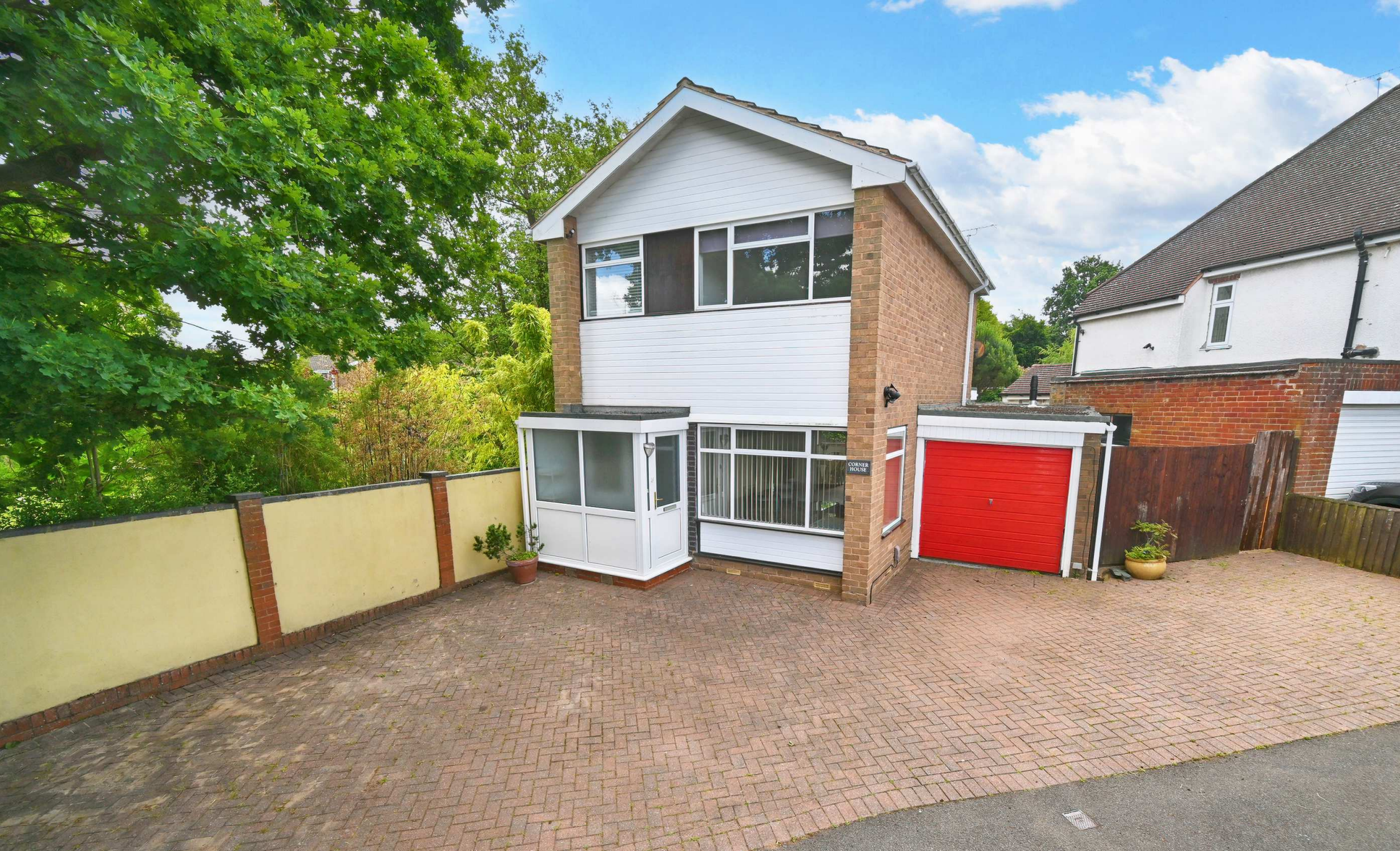
Corner House, York Gardens, Finchfield
