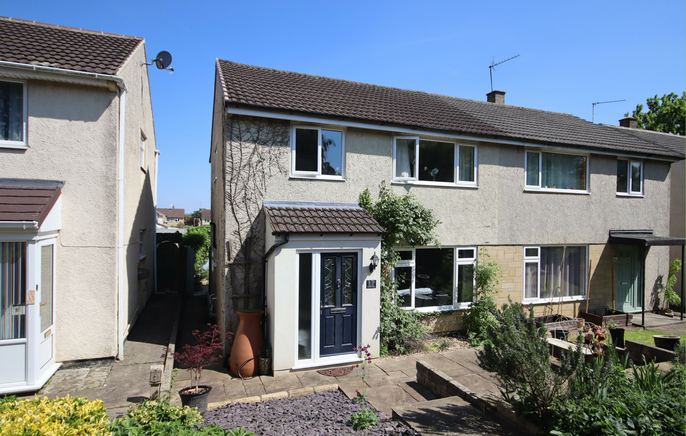
17 Silbury Close Chippenham
