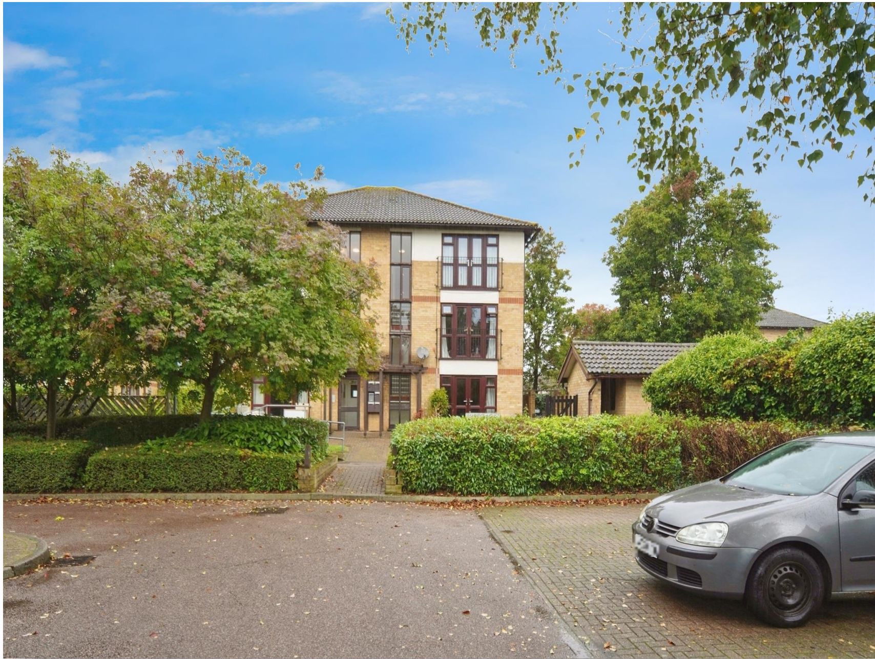
Ashridge House, Chenies Way, Watford, WD18 6UW
