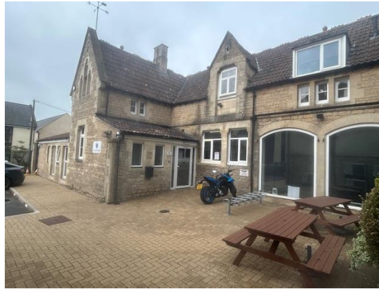
Main entrance door with external bicycle racks and external seating area
