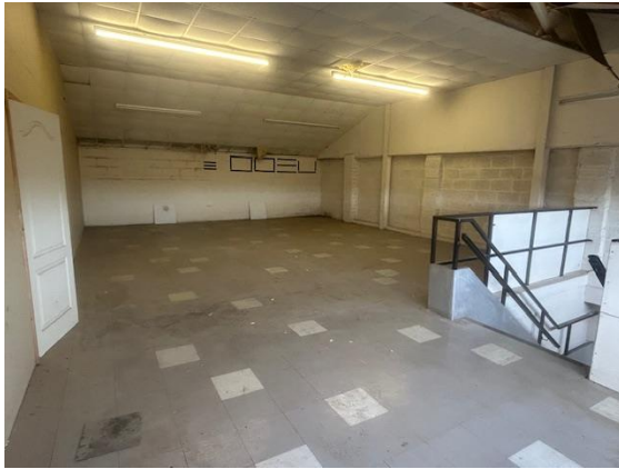
Rear of first floor with fire escape exit
