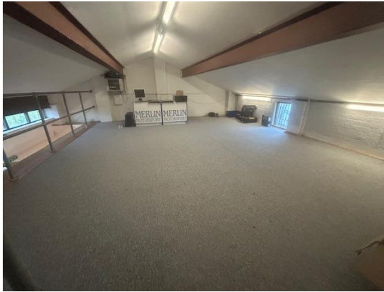
Unit 1 mezzanine floor area
