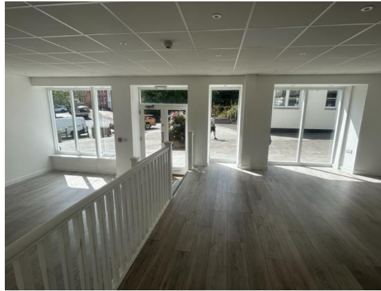
View from rear toward High Street frontage
