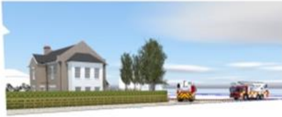
2 View from rear of Dove House
