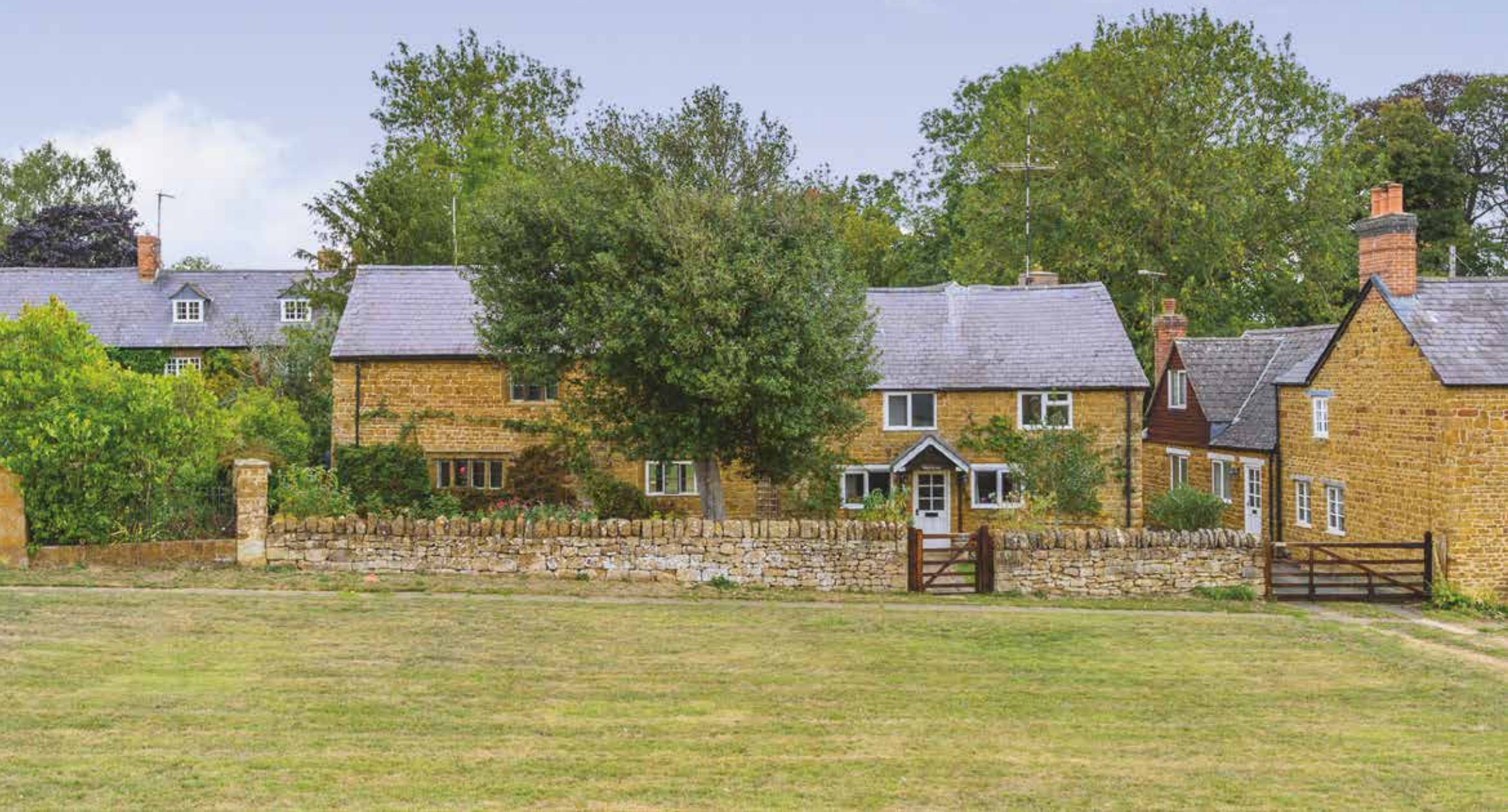
Holly Cottage The Green | Warmington | Banbury | Oxfordshire | OX17 1BU
