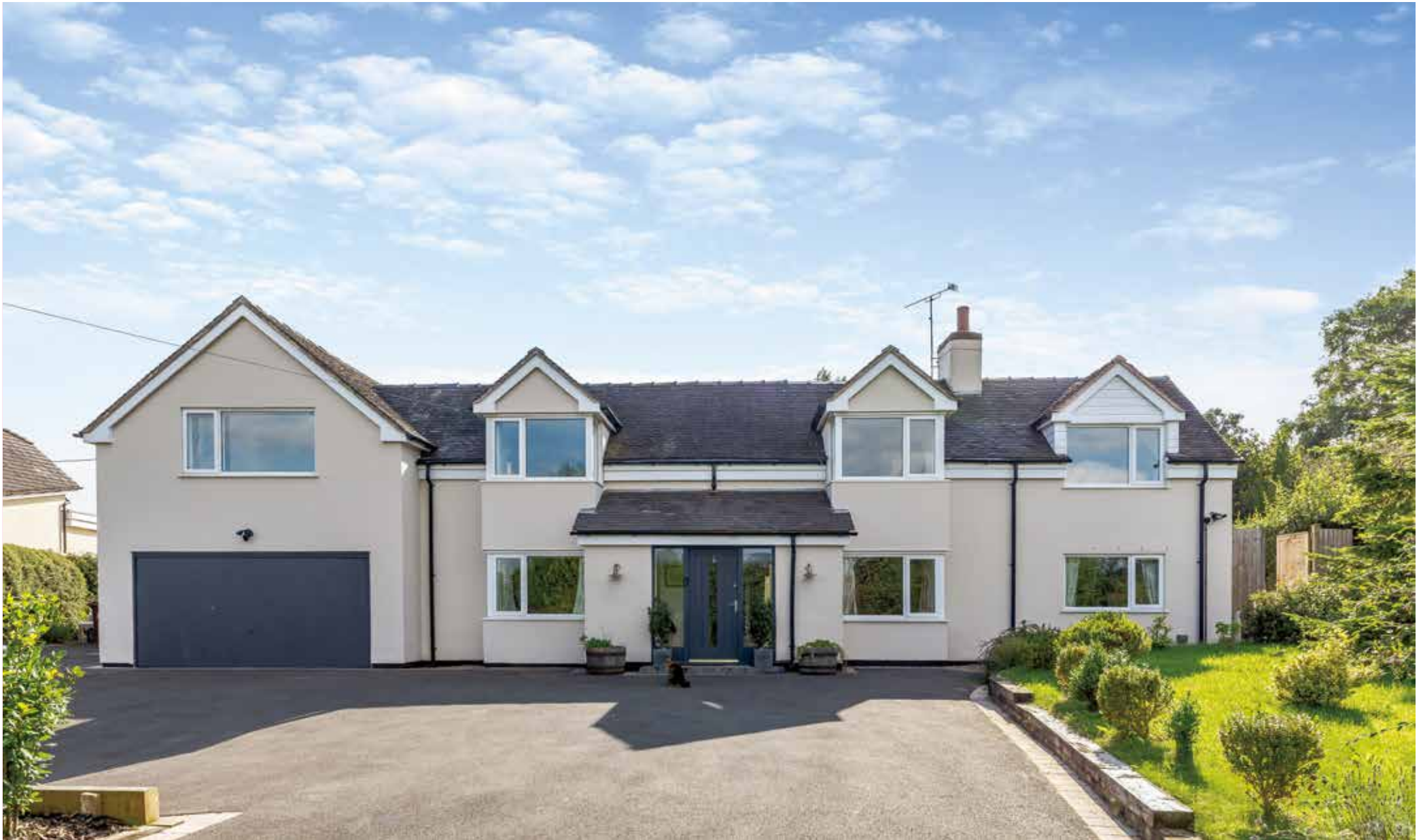
Marlpit Cottage Denstone | Staffordshire | ST14 5DH
