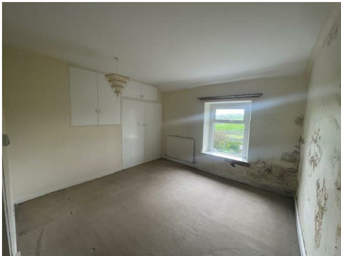
With built in storage and two radiators.
