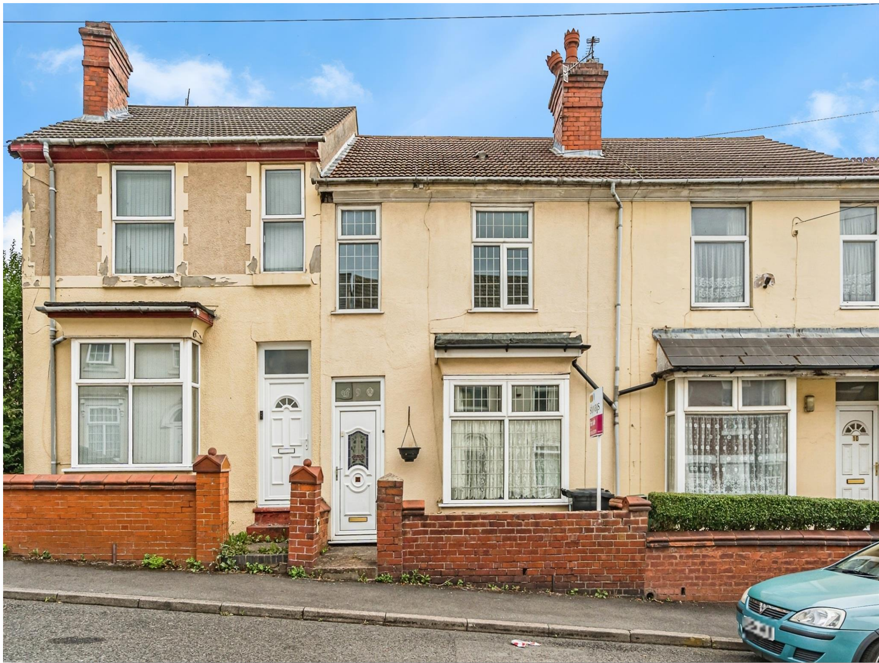
Churchfield Street, Dudley DY2 8QU
