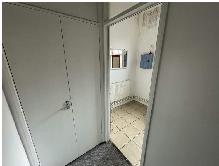
INNER HALLWAY 5'5" x 3'5" (1.657 x 1.061) Built in cupboard housing the water tank.
