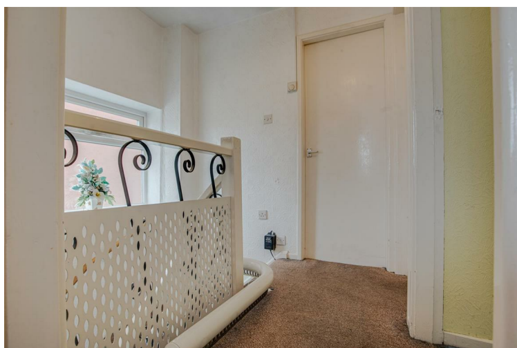
FIRST FLOOR LANDING
