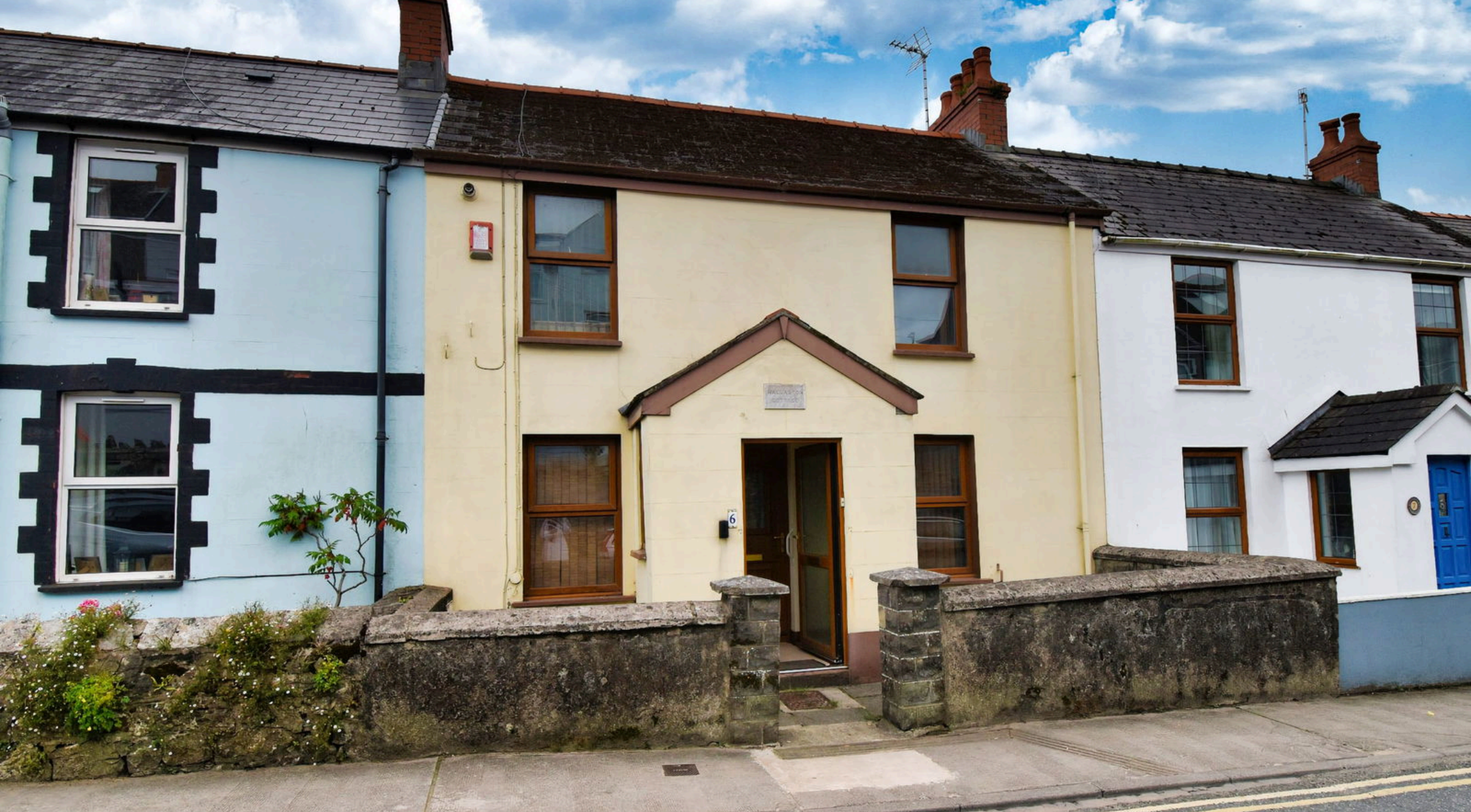
Walleston Cottage, 6 Park Road, Tenby
