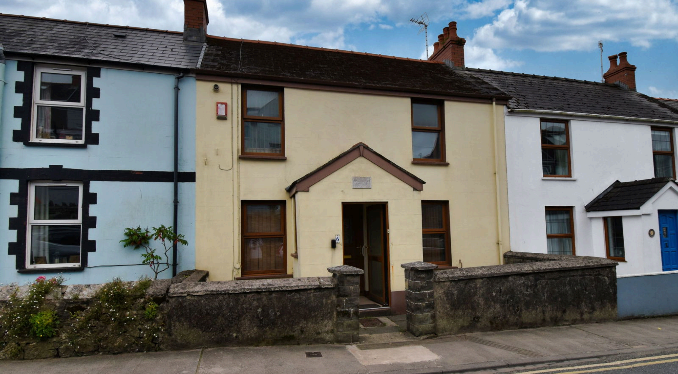
Walleston Cottage, 6 Park Road, Tenby
