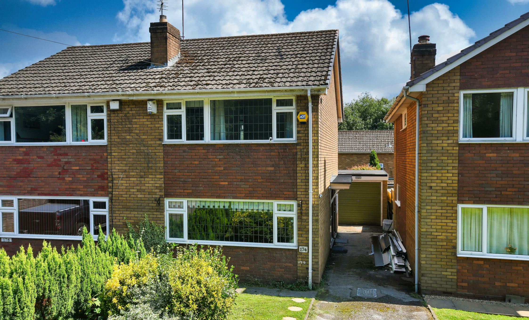
174 Henwood Road, Tettenhall, Wolverhampton, WV6 8PA
