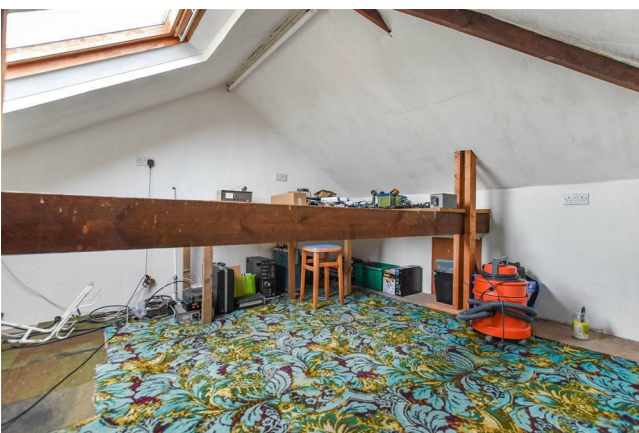
Boarded Loft Space 10'0 x 11'0 (3.05m x 3.35m)
