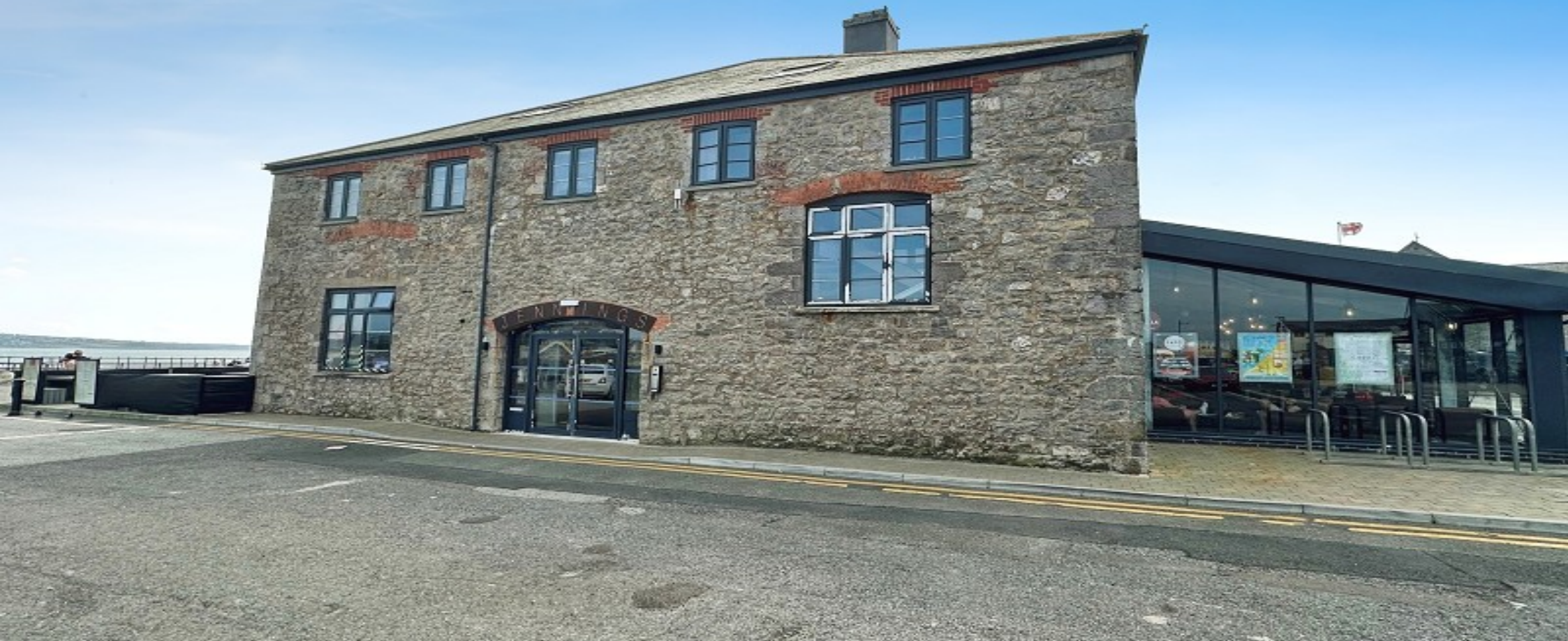
The Jennings Building, The Harbour, Porthcawl. CF36 3XA
