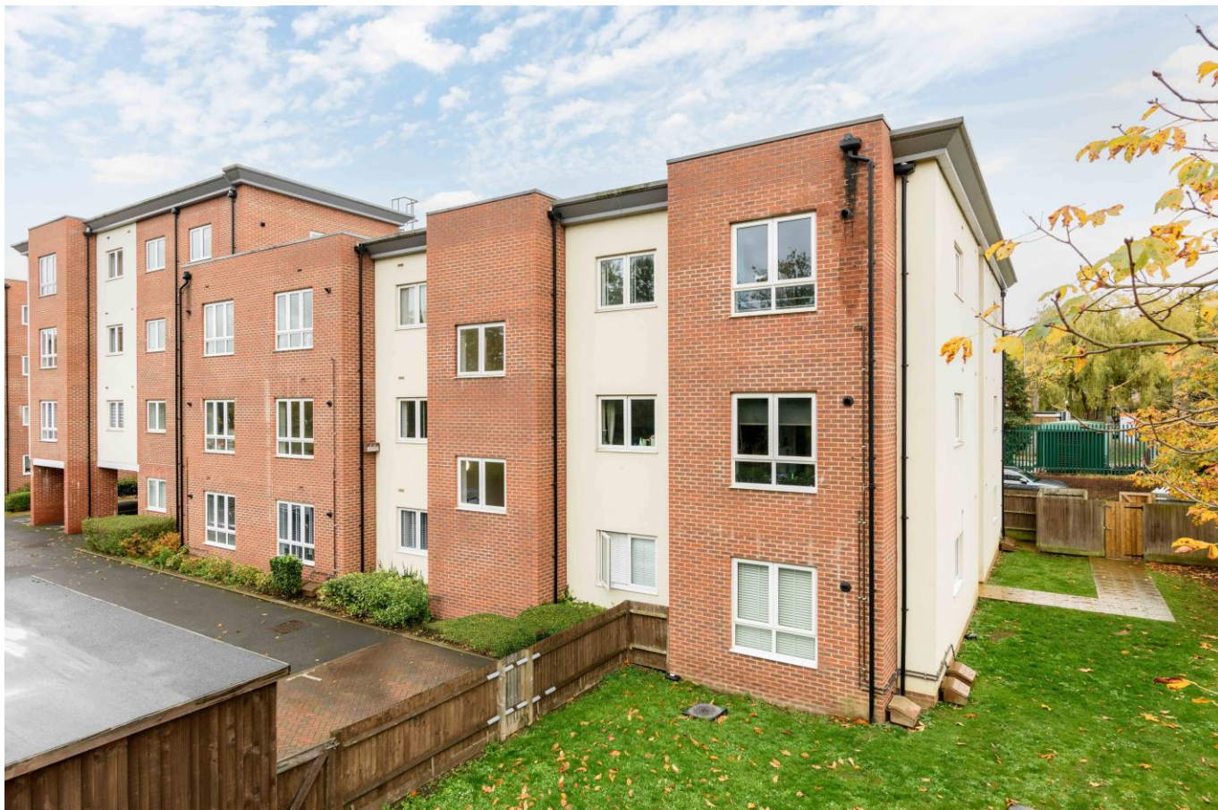
11 Waterloo Court Mayfield Road Hersham Walton-On-Thames Surrey KT12 5AD
