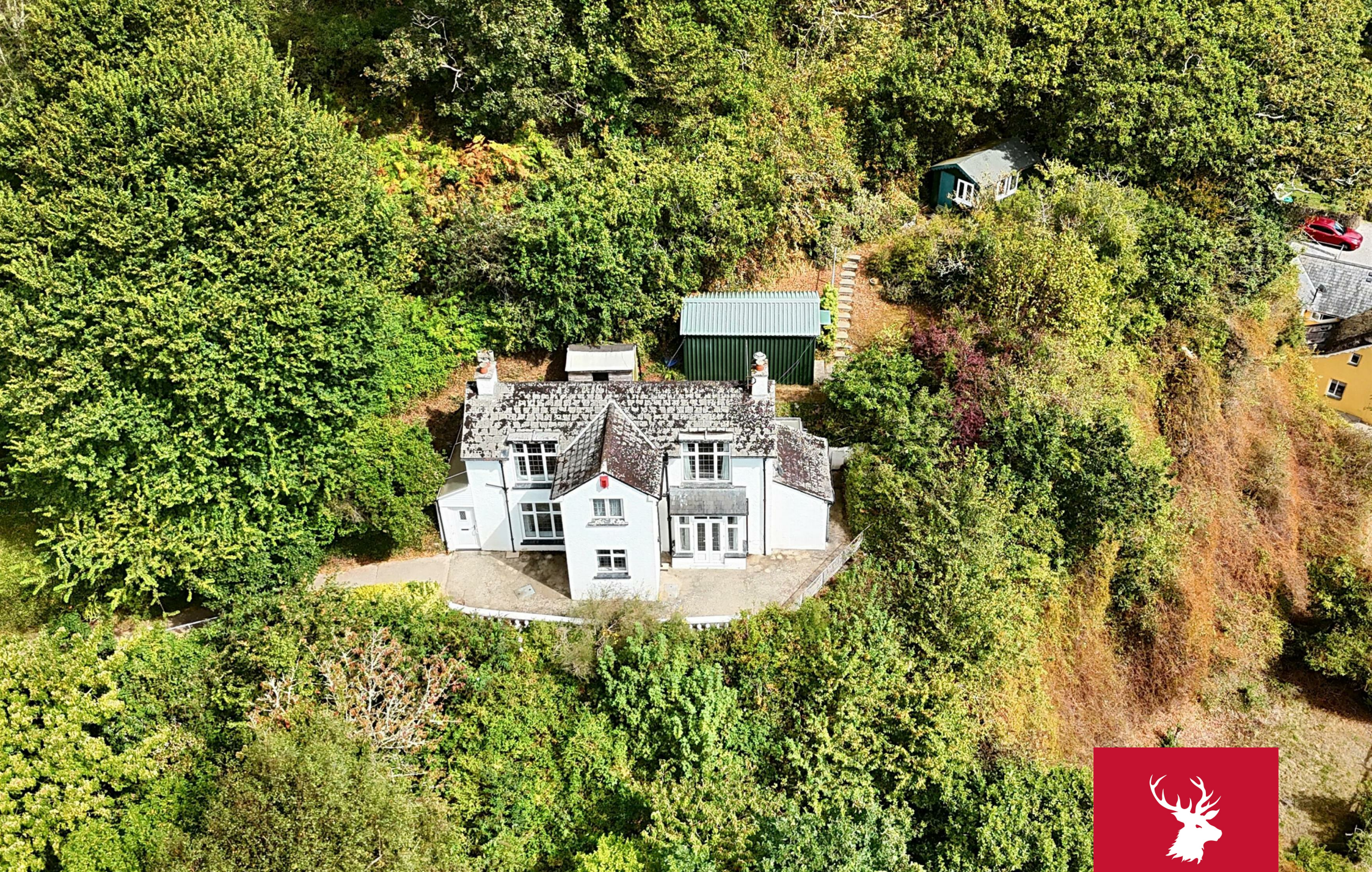
Wall Garden Cottage
