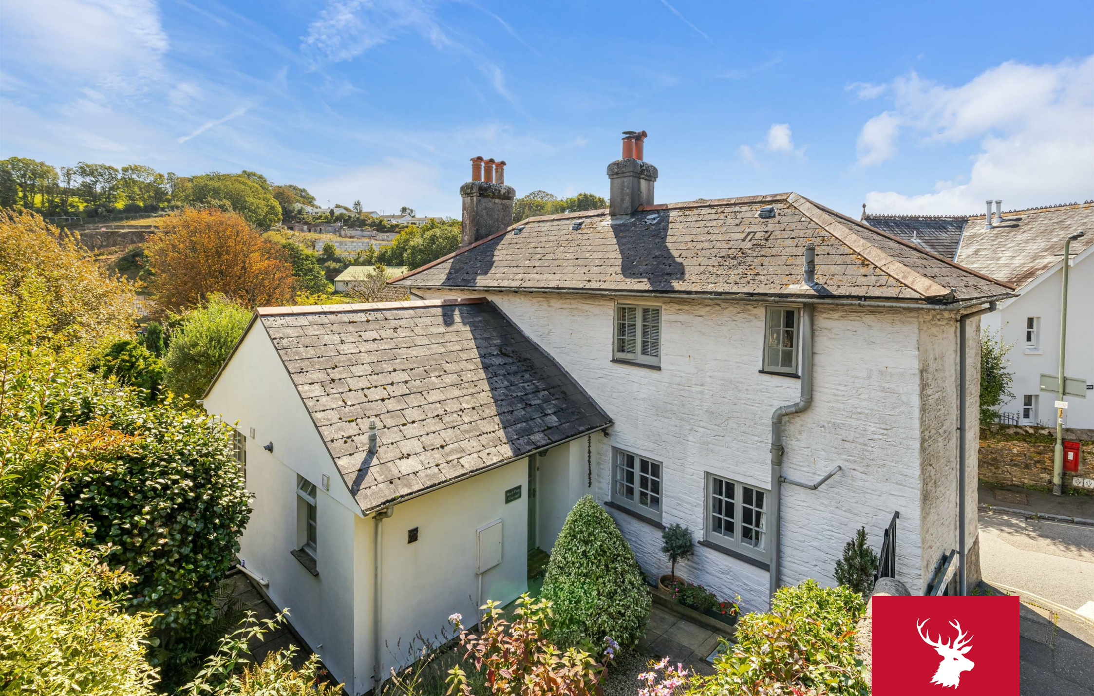
Rack Park Cottage
